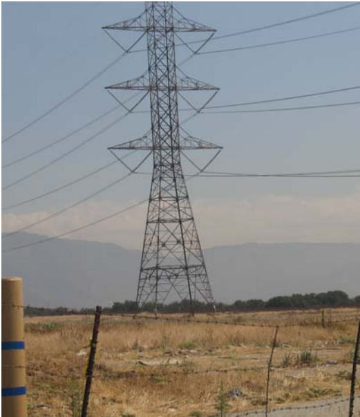
Steel tower along northwestern boundary
