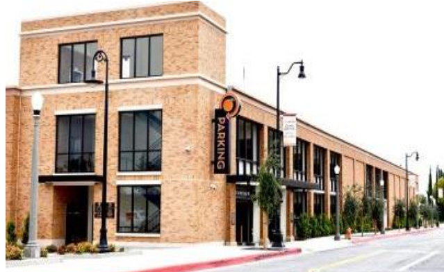
Incorporate architectural elements specific to the Specific Plan area in parking structures.
