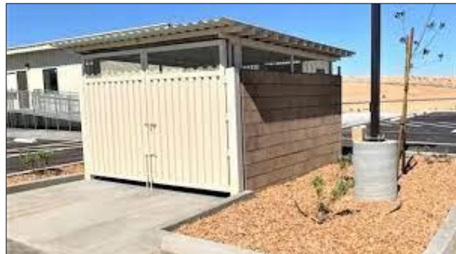
Design trash enclosures walls to be roofed and enclosed, with access by pedestrian gate.
