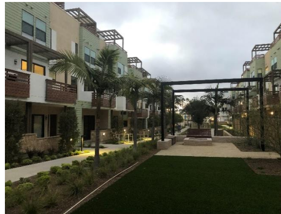
space, walkways, and common open spaces.
