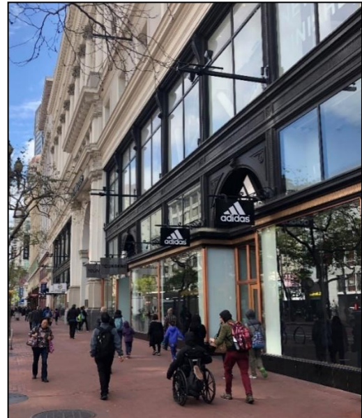
Delineated entrances with articulation, color and material changes, and architectural detailing such as arches.
