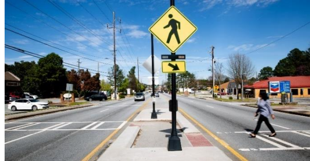
Mid-block crossings provide safe street crossing conditions for pedestrians and encourage cars to slow down.
