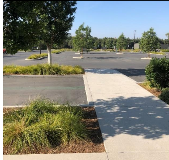
Raised pedestrian walkways create a safe environment when walking through parking lots.
