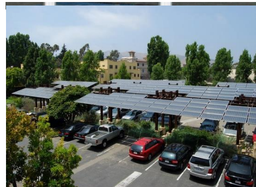
Design shade structures to take advantage of solar opportunities and the reduction of heat island effect.
